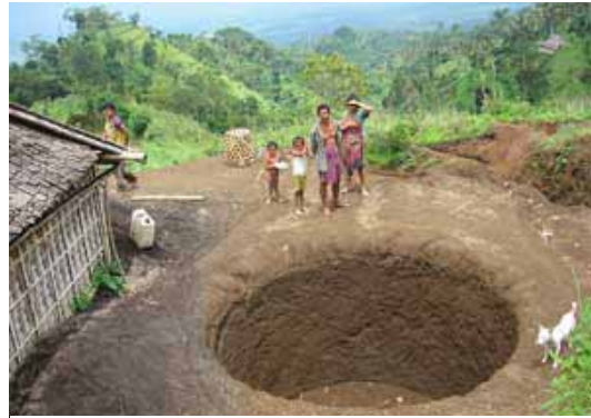
Eager family with 2 infants observing progress of their first home water storage reservoir
