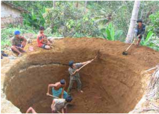
Jatituhu neighbours energetically digging to finish the first cubang excavation
