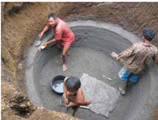
Jatituhu community working together to build the cubang whilst the rain holds off
