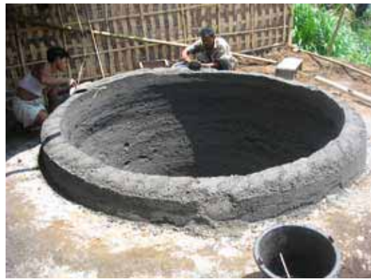
Local men finish cubang walls, ready for the roof
