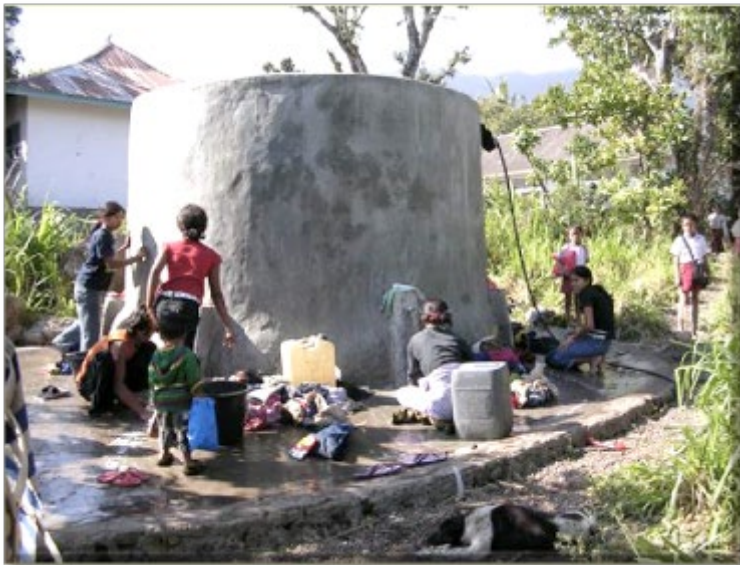
Community reservoir for 400 families from Mt Agung spring (finished 11 2004)
