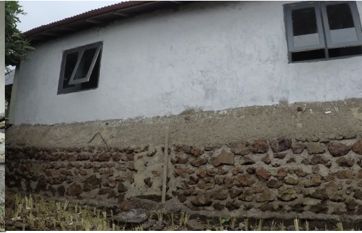
Rebuilt, with reinforced concrete retaining wall
